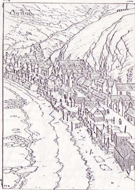
Fig. 2 - Sea wall built by individuals. Sea energy was spent on beach and between piles.
