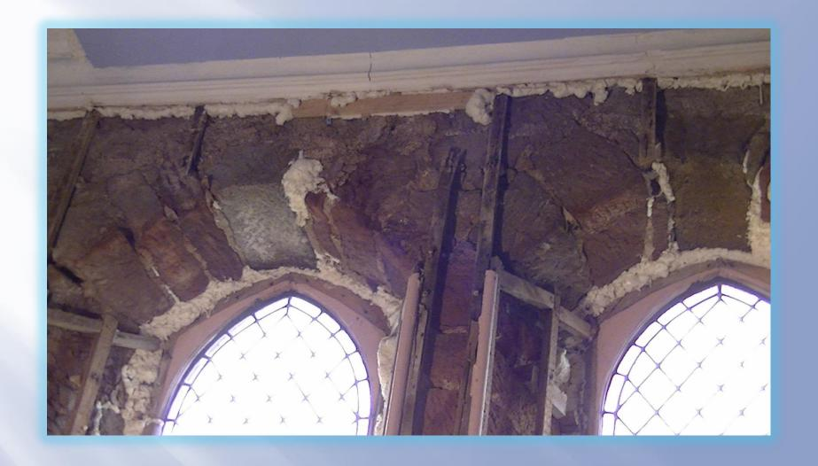
The upstairs windows were falling out (during the winter of 2013-14 they had to be propped up inside with a pole tied to the end of a pew!) They were fixed back to the stone with metal straps then sealed off with expanded foam inside and silicone sealer outside.
