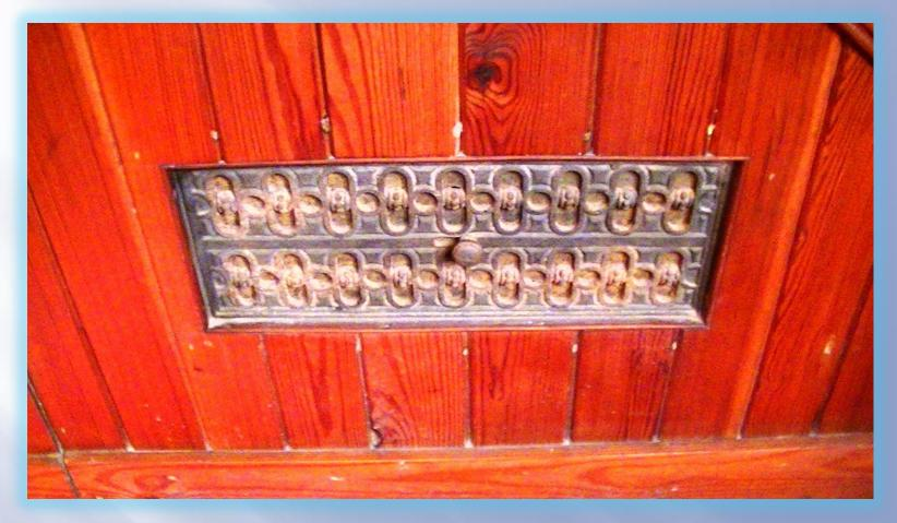
Looks like a ventilator on the side of the pulpit but it's actually connected by a wooden duct to a heating chamber below the church. It's unclear what sort of fire they used because the chamber is partially bricked up. It would seem to have been pretty basic though – just a big fire with the heat rising by convection up through the church. Apparently it was never a success because it channelled up smoke as well as heat!
